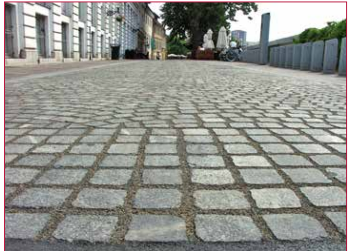
Die fertig verfugte und trittsichere Fläche | The completed surface – clean joints and firm under foot | Zalita površina za zanesljiv korak
